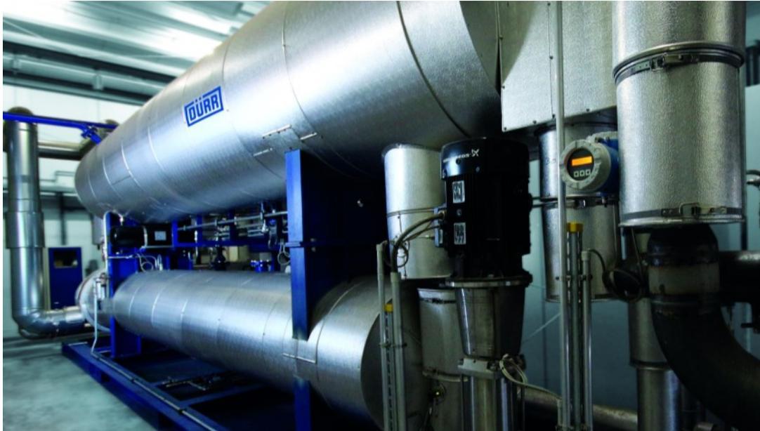
Figure 1: Heberndorfer Leistenfabrik converts waste products into electricity and heat energy with a high level of efficiency using an **Eco+Energy** ORC system from Dürr Cyplan.
